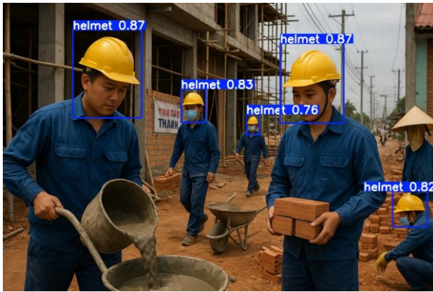
Figure 7. Experimental results on a construction site
